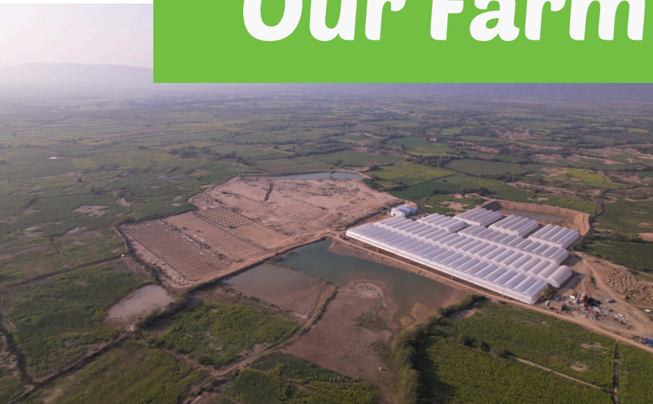
Lakheri - 24 Acres Partially under Construction
