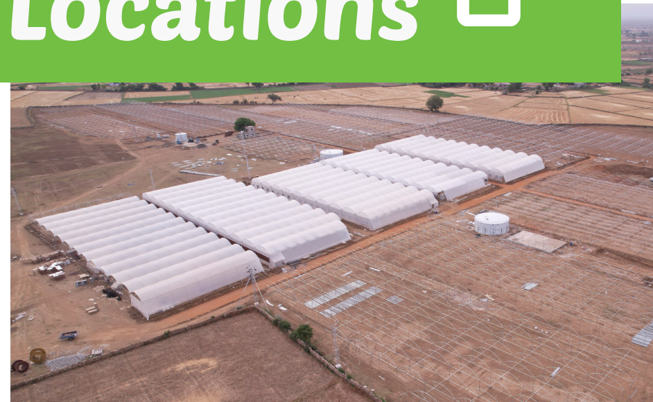
Namana - 25 Acres Under construction
